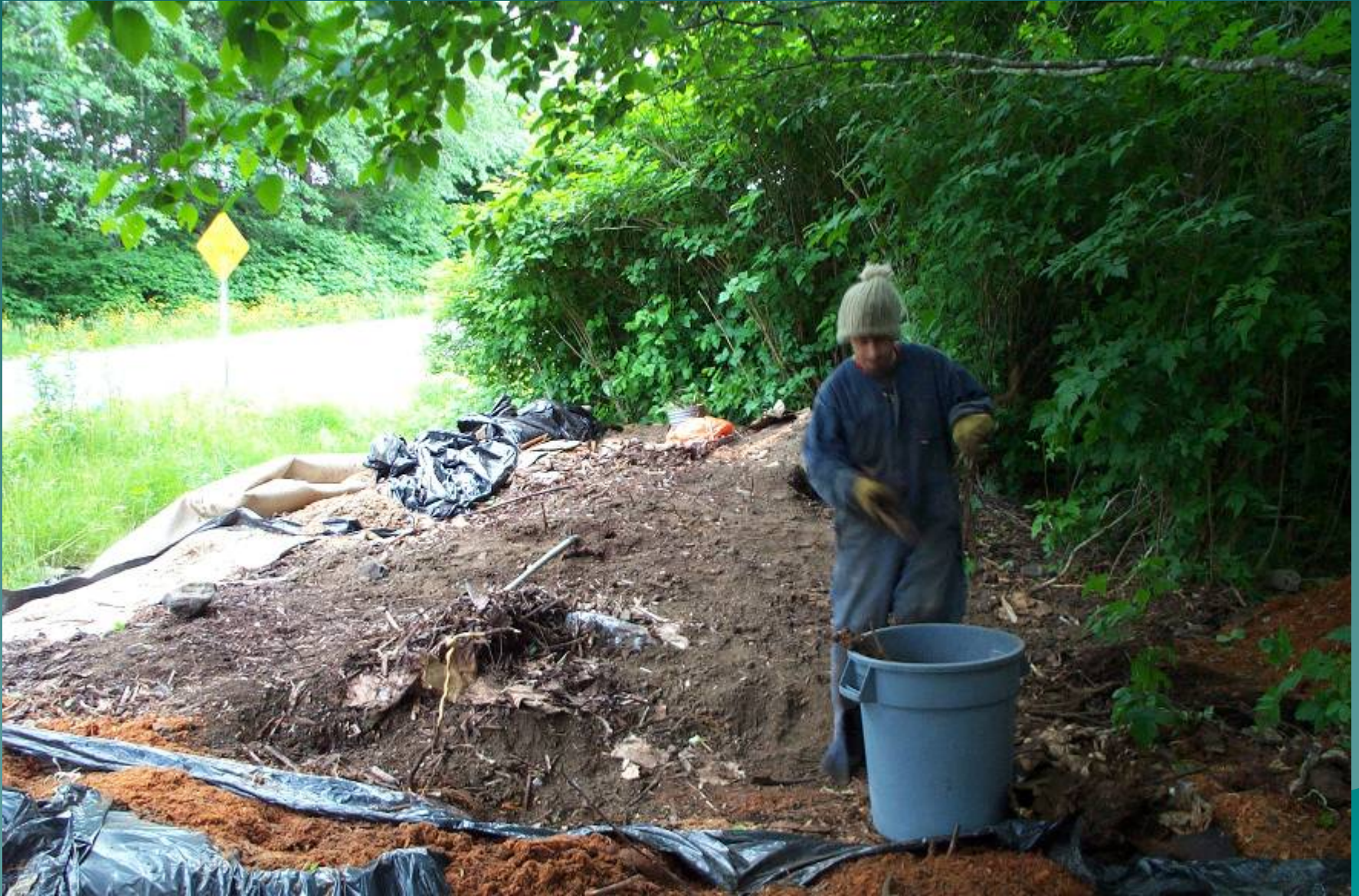
Preparing site for Phase 3: Introduction of native vegetation.
