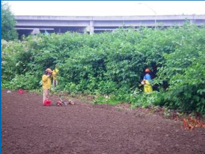
Before control, starting to cut
